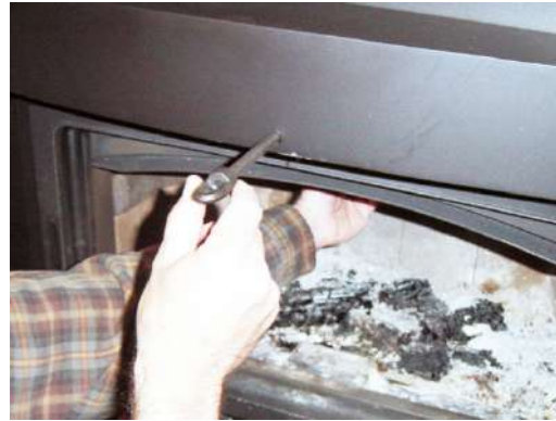
Figure 24: Attaching the extension rod
