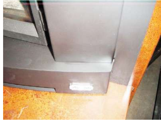
Figure 18: Face aligned flush with the insert
