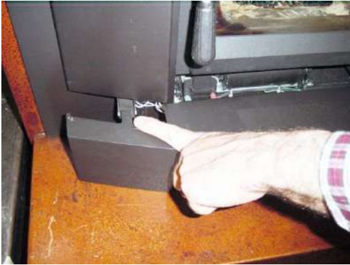
Figure 17: Attaching the lower face
