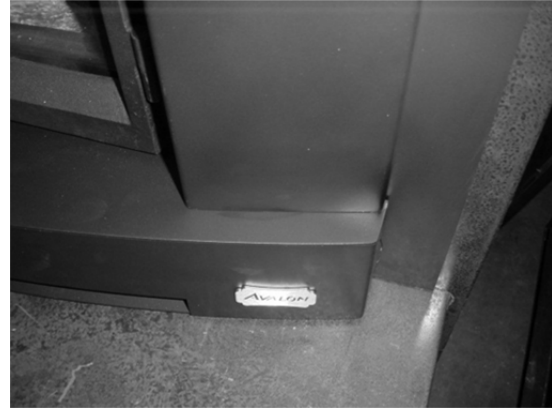
Figure 18: Face aligned flush with the insert
