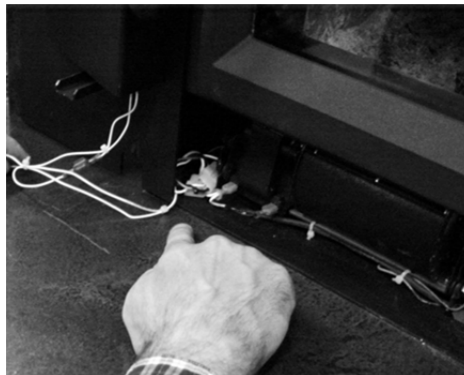
Figure 11: Tuck excess wires
