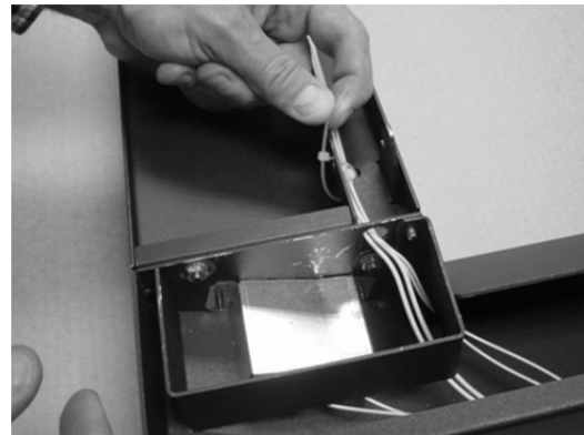
Figure 6: Securing the lock-tie
