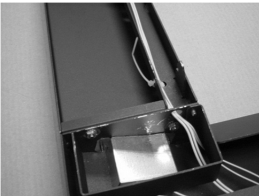
Figure 7: Wires secured with lock-tie
