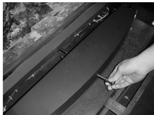
Figure 22: Tightening the air control rod
