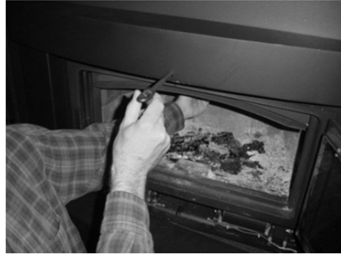
Figure 24: Attaching the extension rod
