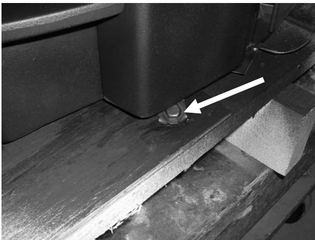
Photo 1 – Pallet Mounting Clip Detail (Right Front Shown - Façade Installed)
