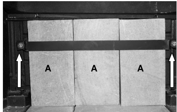
Photo 14 – Install & Secure Firebox Rear Stones
